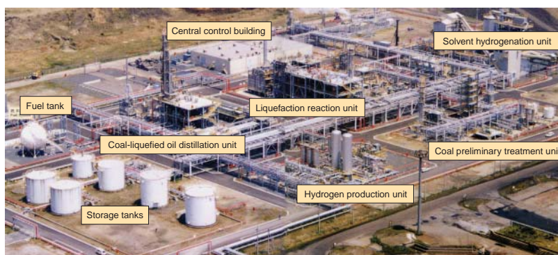
Fig. 3 NEDOL Process pilot plant (150 t/d)
